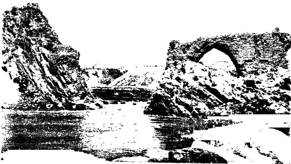
75. RUINED BRIDGE ACROSS SAIMAREH AT SEFALEH, HULAILĀN
